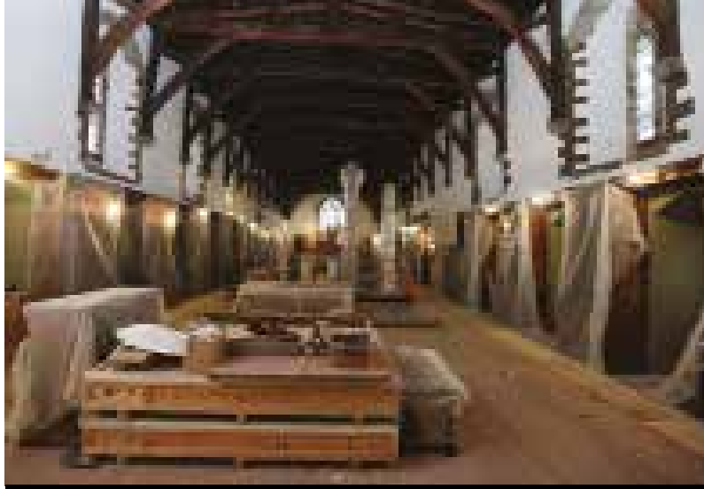
BEFORE: The Monk's Dormitory in progress March 2015.
