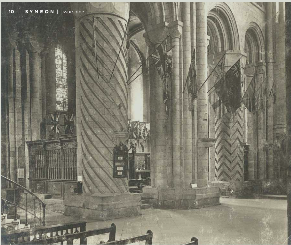
Internal View of the Durham Light Infantry Memorial Chapel, 1925', DRO, D/CL 5/761. Durham County Record Office. Reproduced by permission of Durham County Record Office.
